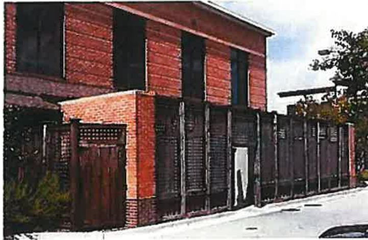
Figure 6-5-9: Screening elements integrated with the building
